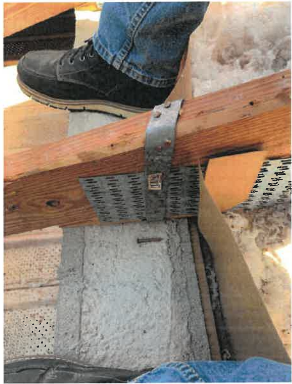
Figure 24: Roof to wall attachment.
