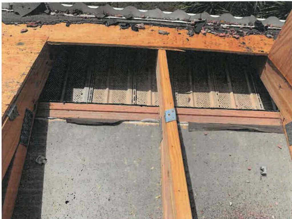
Figure 34: Roof to wall attachment.
