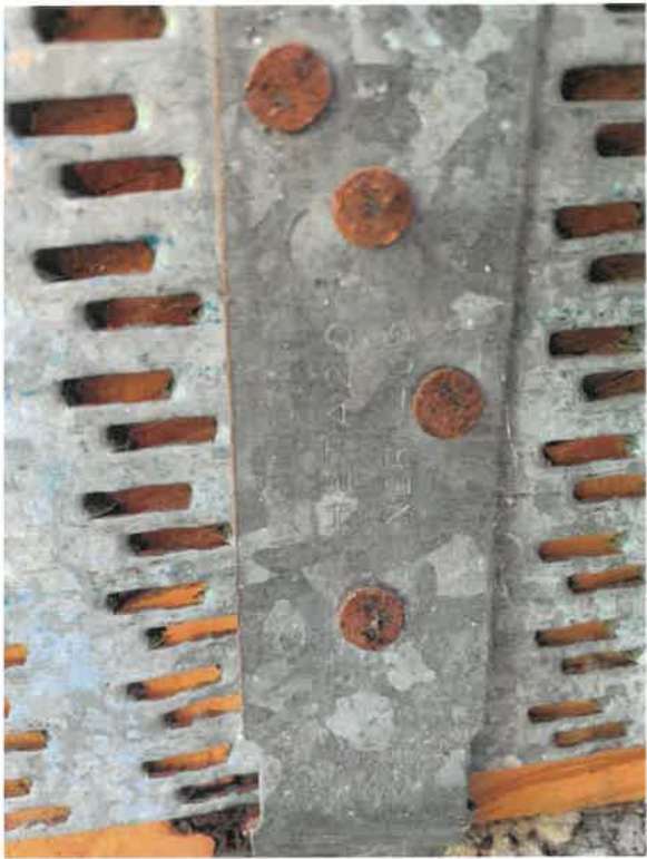
Figure 26: Roof to wall attachment.
