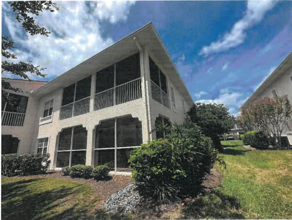
Figure 19: South / East Elevation.
