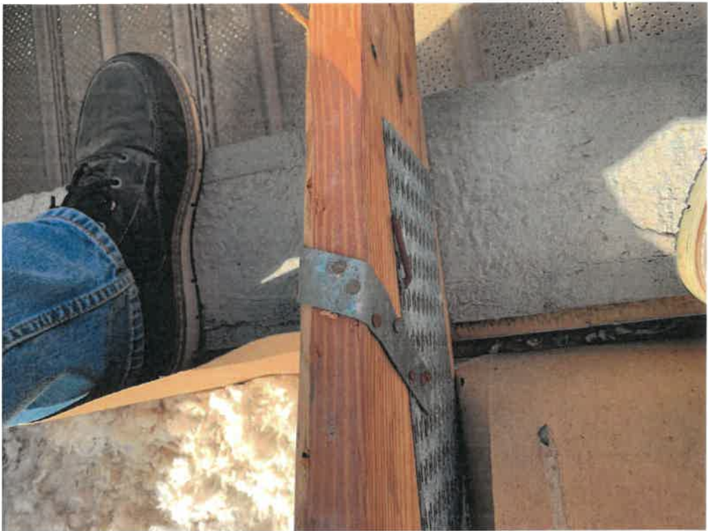
Figure 25: Roof to wall attachment.
