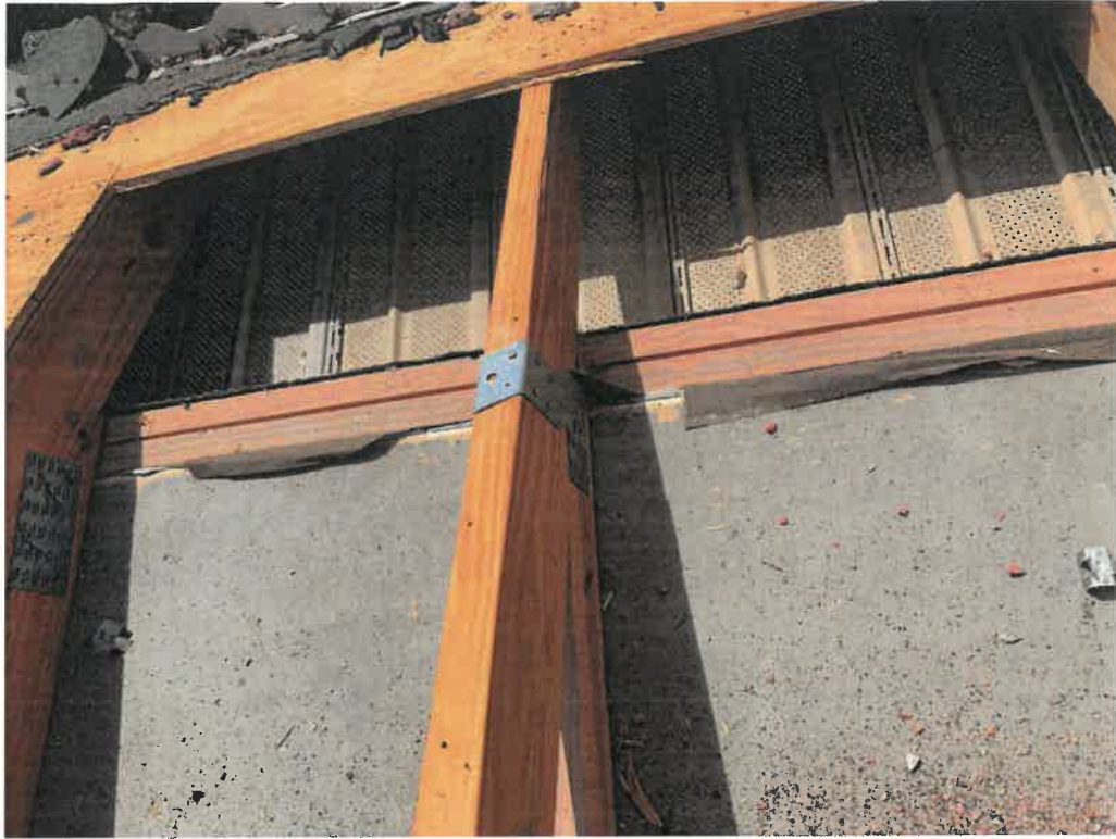
Figure 35: Roof to wall attachment.
