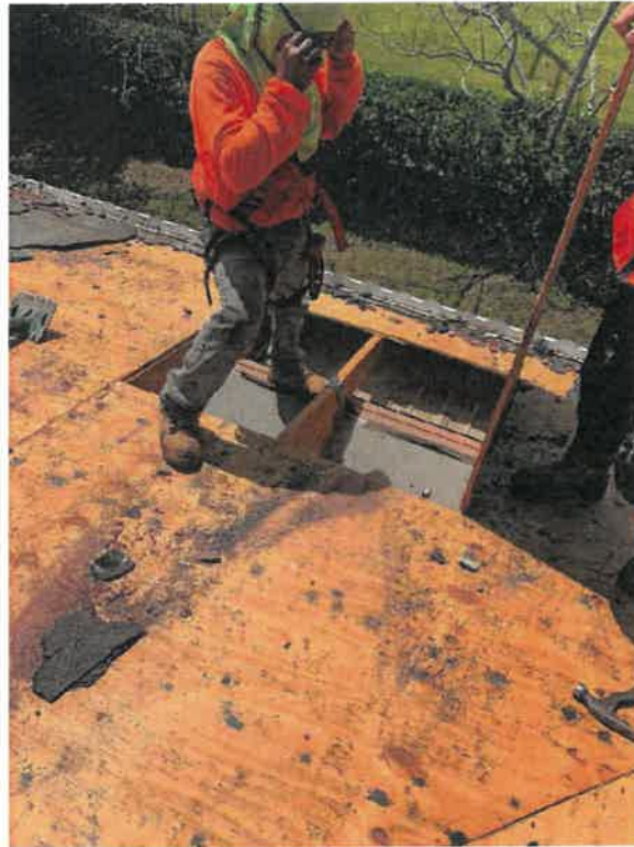
Figure 33: Roof to wall attachment.
