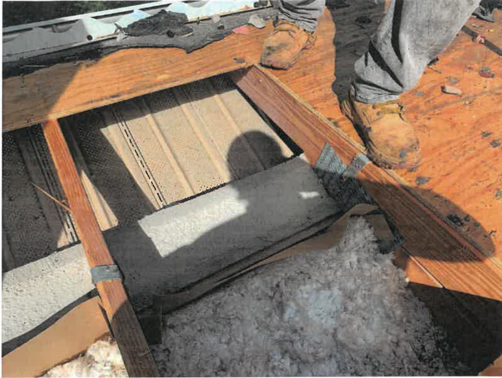
Figure 27: Roof to wall attachment.
