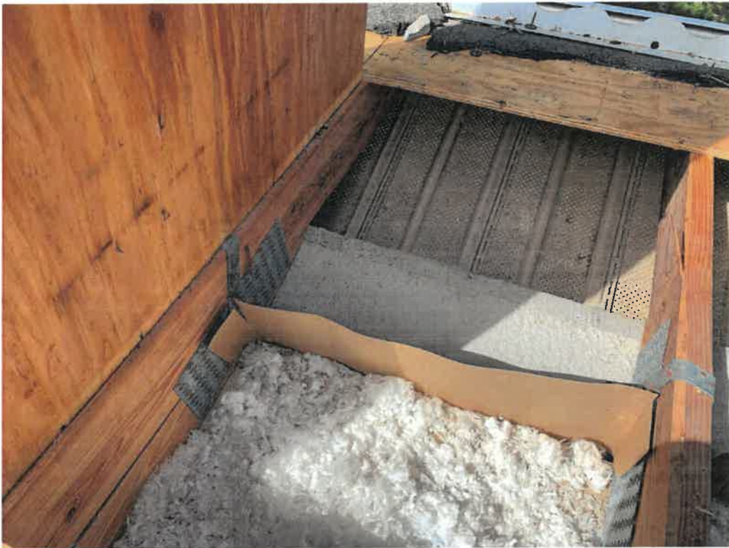
Figure 28: Roof to wall attachment.
