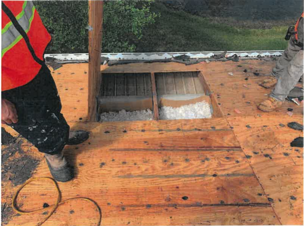
Figure 23: Roof to wall attachment.
