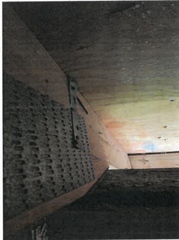
Figure 29: Roof to wall attachment.
