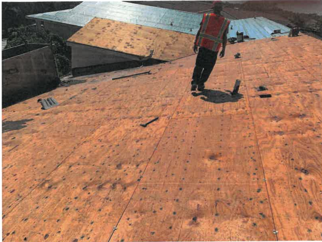
Figure 33: Roof to deck attachment.
