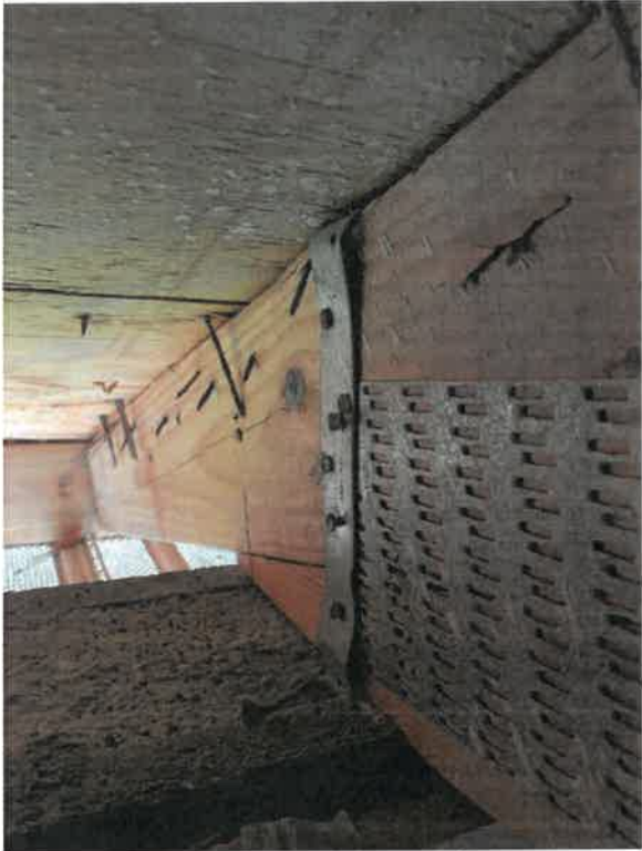
Figure 27: Roof to wall attachment.
