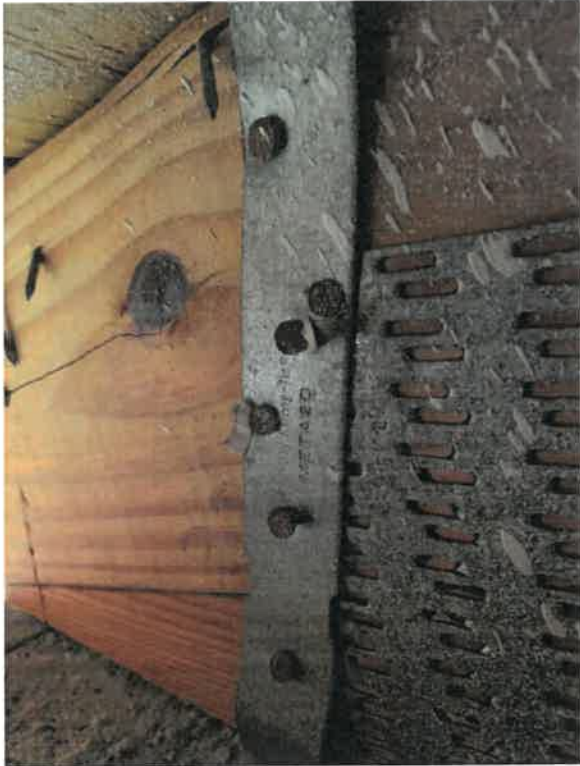
Figure 28: Roof to wall attachment.
