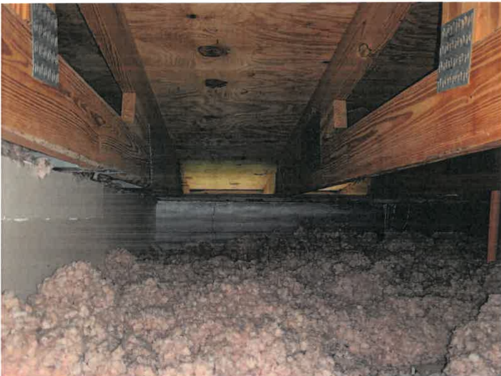
Figure 20: Roof to wall attachment.
