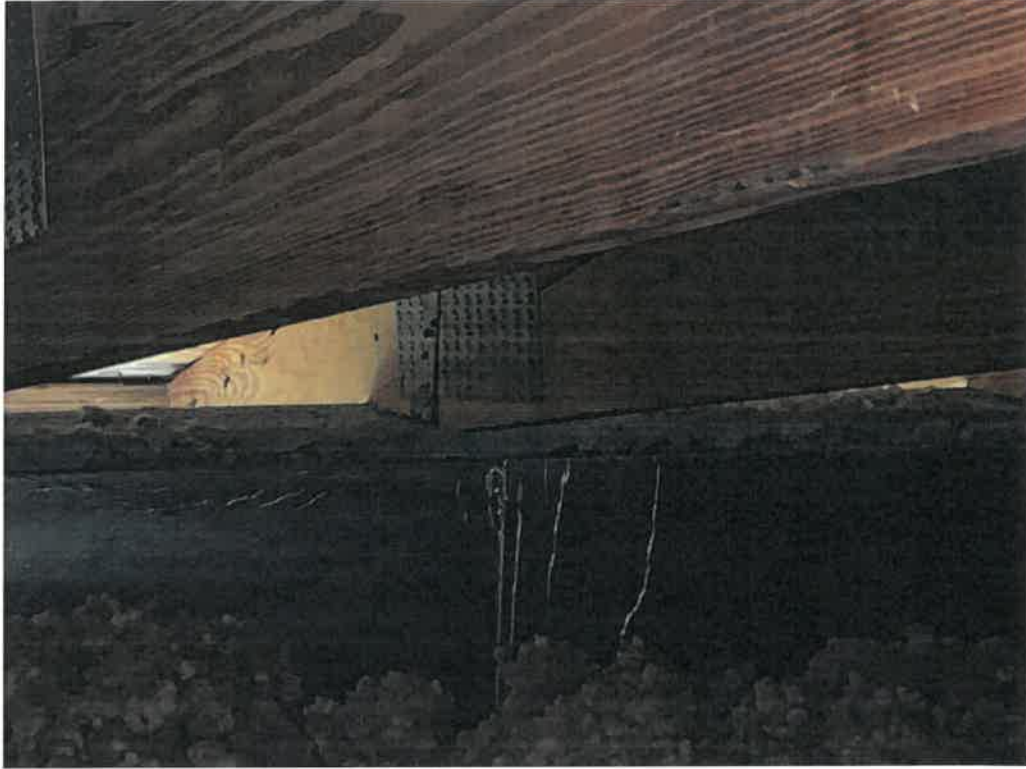
Figure 23: Roof to wall attachment.
