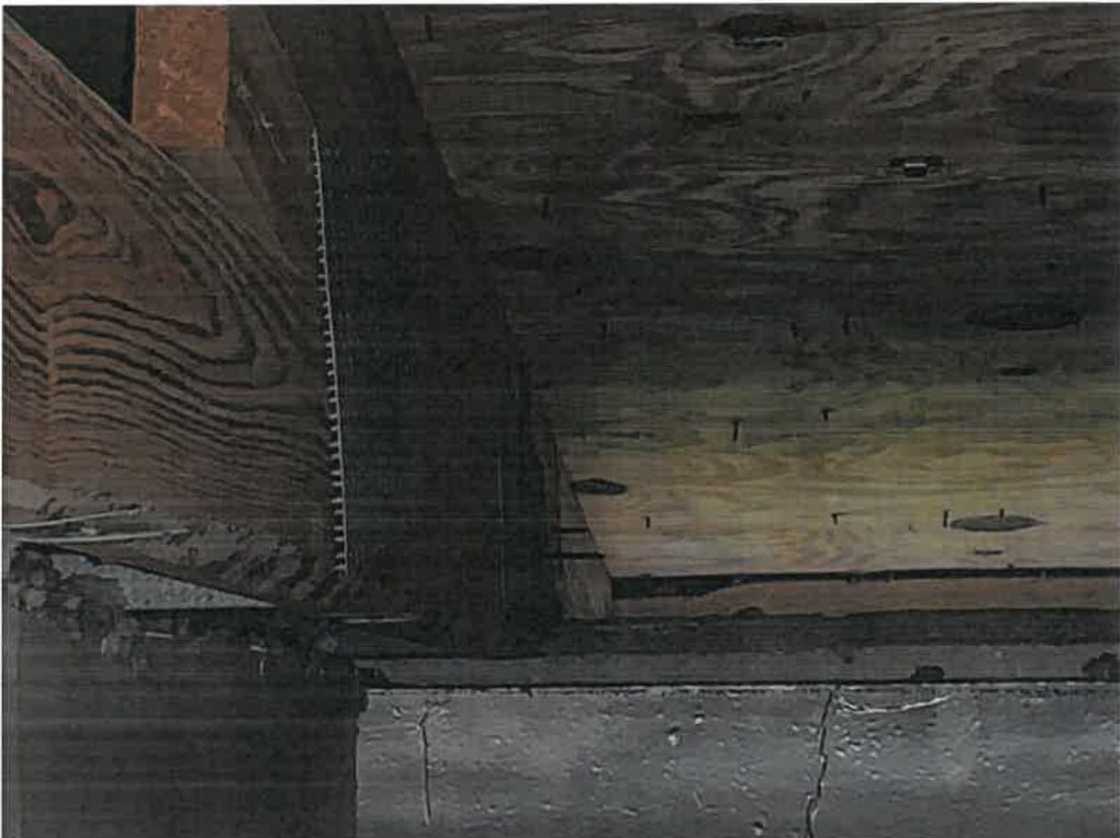
Figure 22: Roof to wall attachment.
