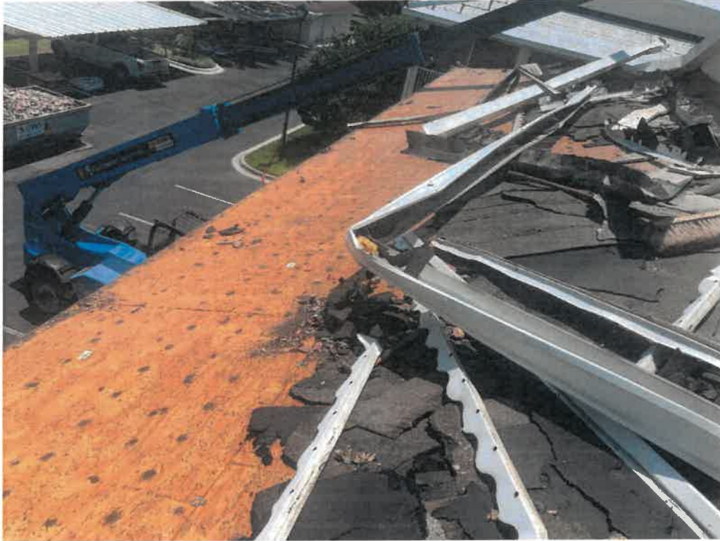
Figure 25: Roof to deck attachment.
