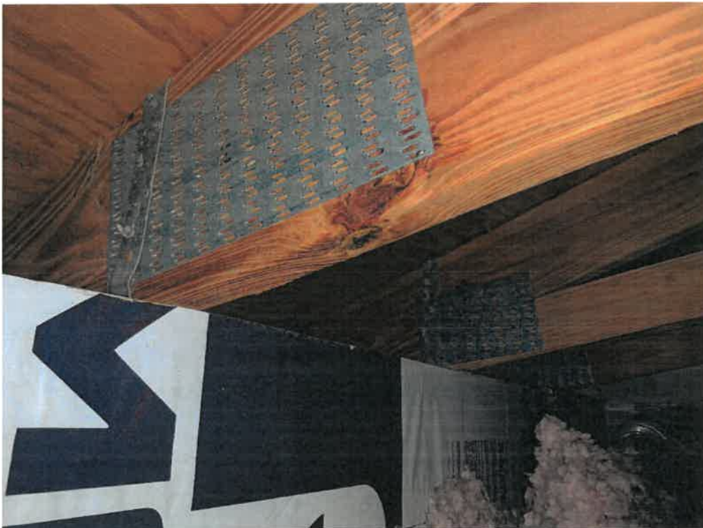
Figure 20: Roof to wall attachment.
