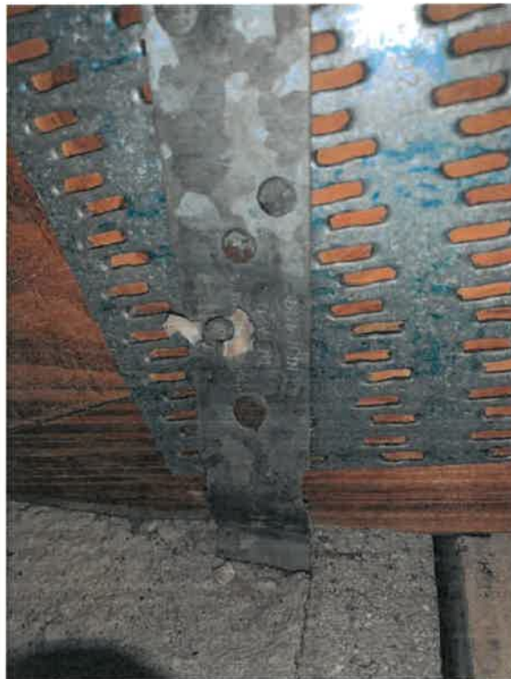
Figure 22: Roof to wall attachment.
