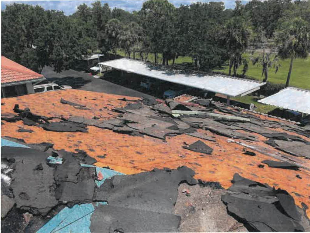
Figure 23: Roof to deck attachment.
