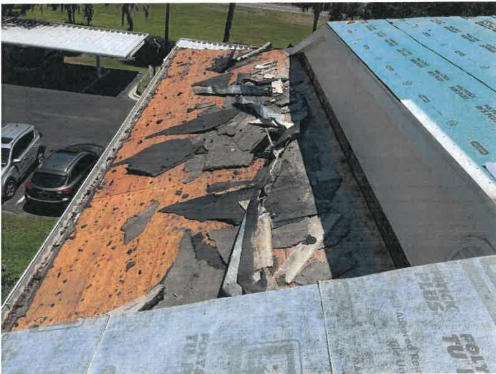
Figure 24: Roof to deck attachment.
