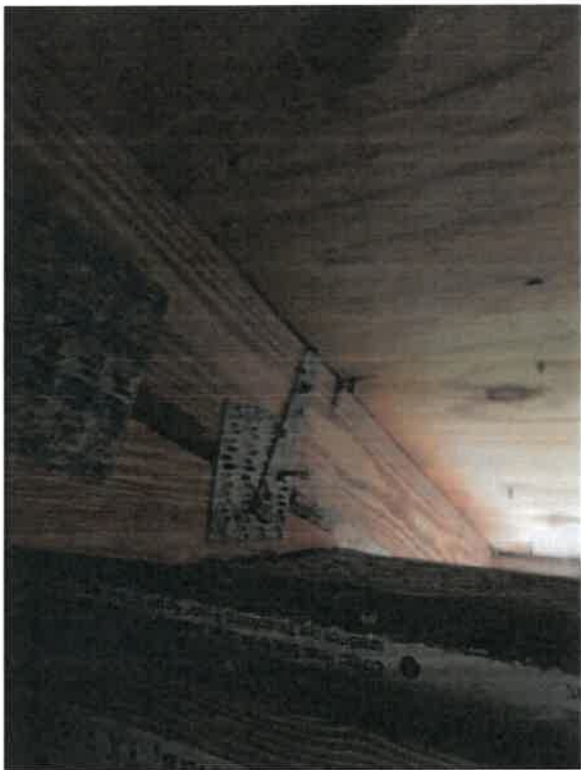
Figure 18: Roof to wall attachment.
