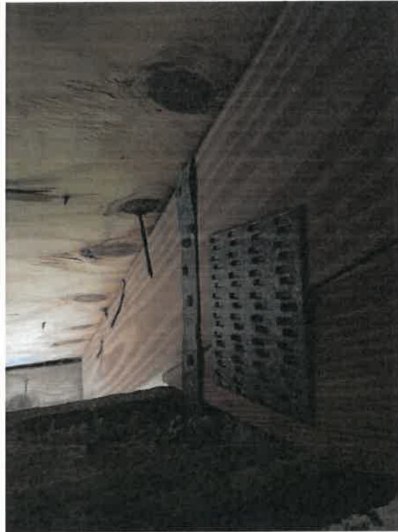
Figure 19: Roof to wall attachment.
