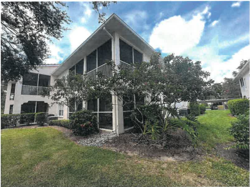
Figure 14: South / East Elevation.
