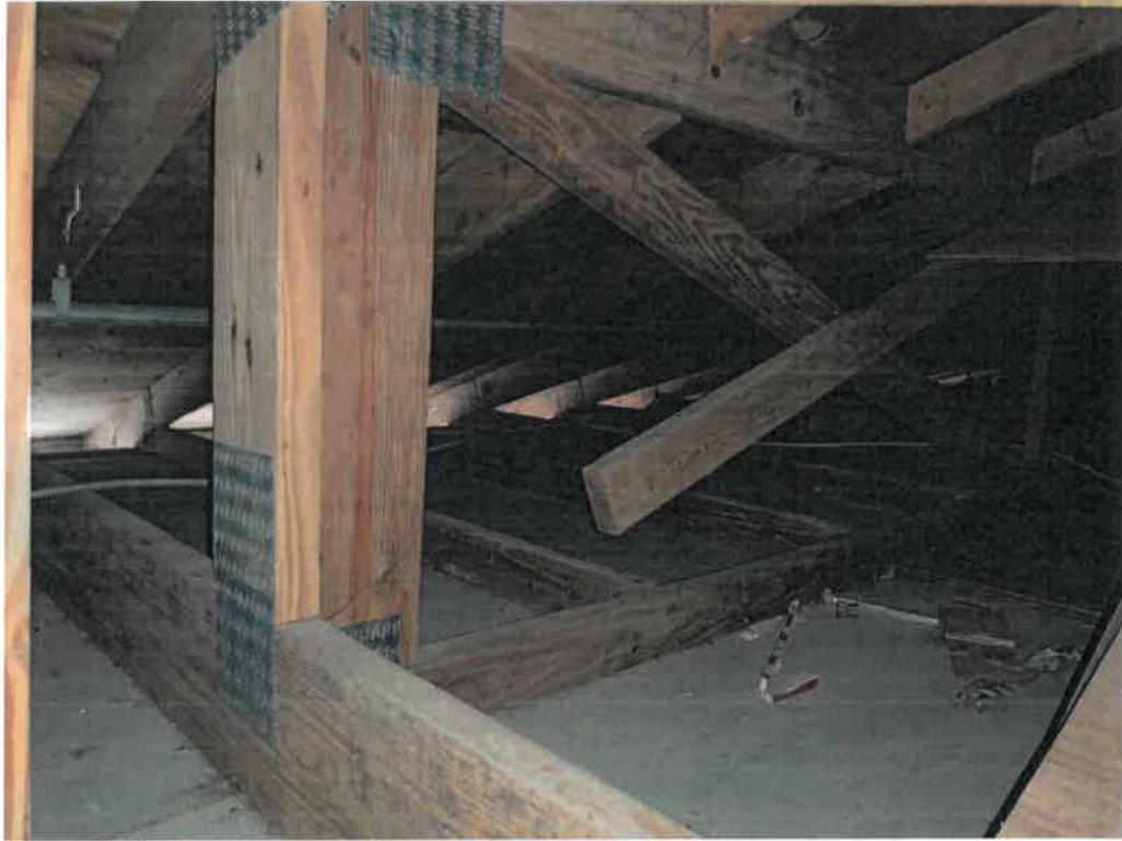
Figure 11: Roof to wall attachment.
