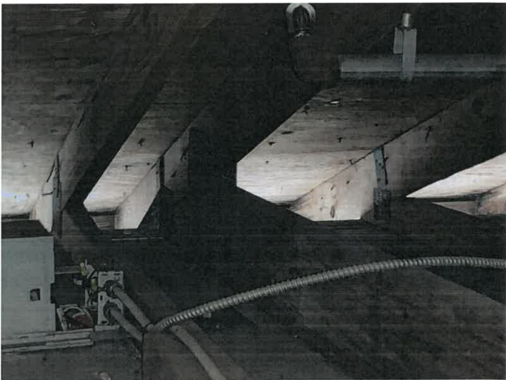
Figure 12: Roof to wall attachment.
