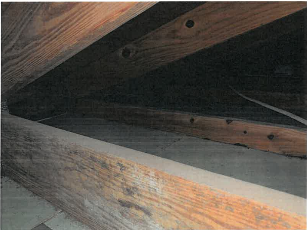
Figure 10: Roof to wall attachment.
