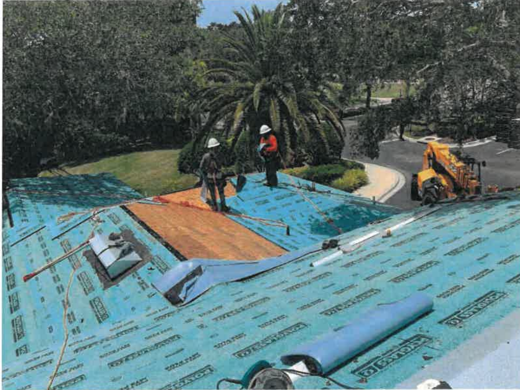
Figure 13: Roof to deck attachment.
